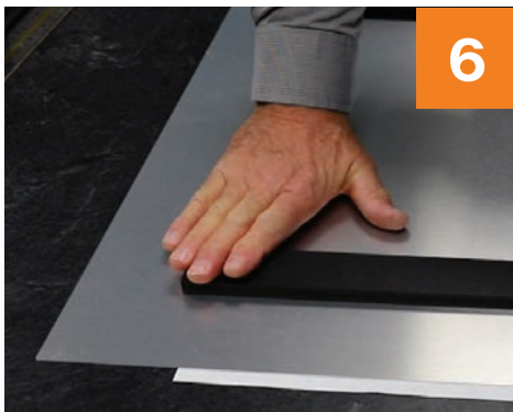
6 Firmly press down on the entire perimeter to ensure full adhesion on all sides.
