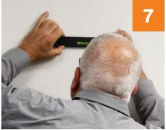
Using the provided leveling wall cleat and a pencil, mark the drill holes in the desired mounting location.
